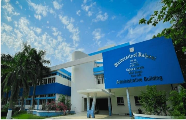
University Administrative Building
